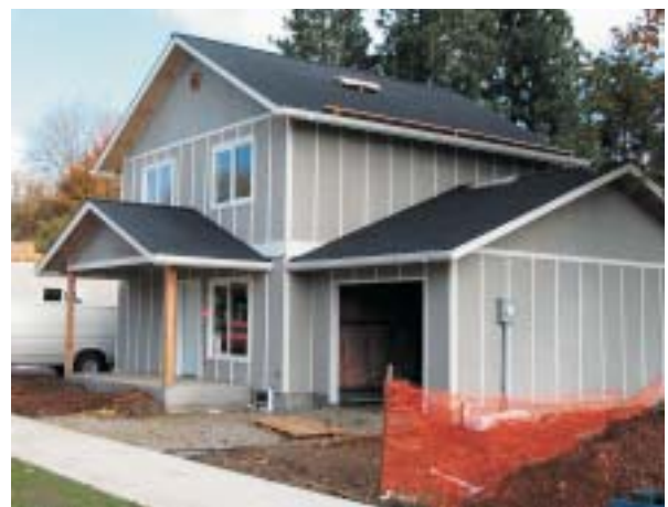
Santa Clara Glen home under construction
