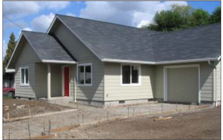
43rd Street Home Under Construction
